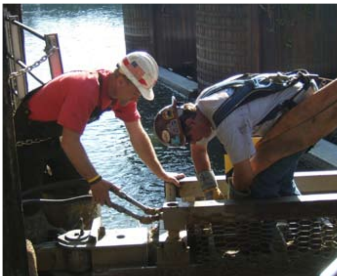
Corps and Triad mechanics work atop the left leaf of Gate 1
